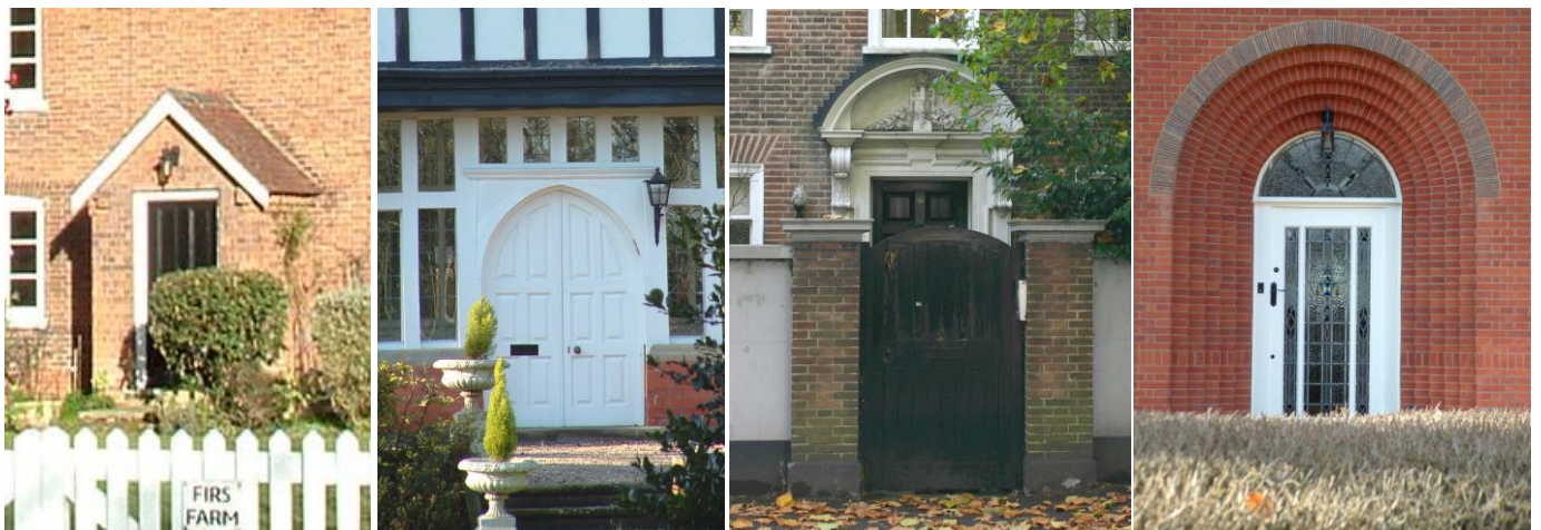
Above from left to right: timber four panelled door and brick porch with pitched roof, six panelled double doors in pointed arch doorway and leaded glazed surround, classical style portico with segmental pediment and six panelled timber door, stepped arch surround and glazed timber door with stained glass detailing and sunburst fanlight.
