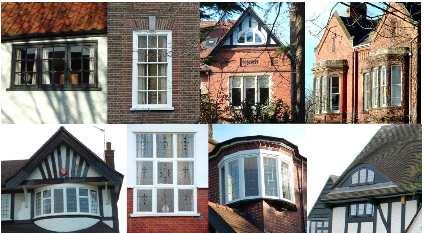
Clockwise from top left: Tripartite timber casement, 15 pane vertical sliding sash, semicircular gable window and stone mullioned casement, a pair of bay windows with vertical sashes and ashlar dressings, eyebrow dormer, circular corner bay with leaded glass timber casements, 9 pane stained glass casement, curved first floor bay window with leaded glass timber casements.
