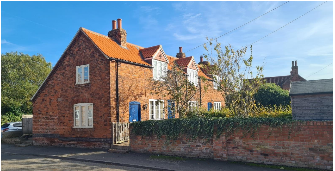
Figure 18 - Inholms Road, opposite the village hall
