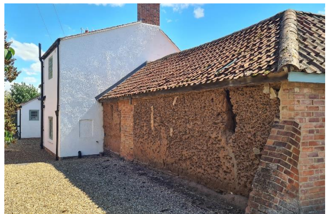
Figure 9 – Mud wall at Smitte Farm, Main Street (Zone 2)
