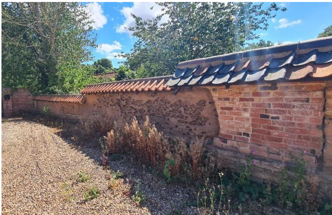
Figure 8 -Mud Wall, Church Lane (Zone 1)
