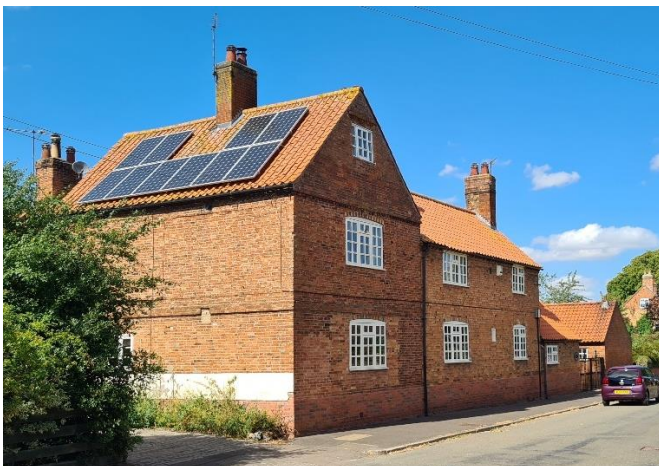
Figure 22 - Hall Farm Cottage, Main Street
