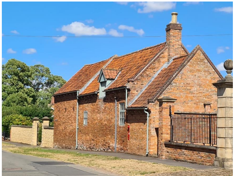
Figure 19 - Stable, Coach House, Blacksmith's Forge and Adjoining Wall, Main Street
