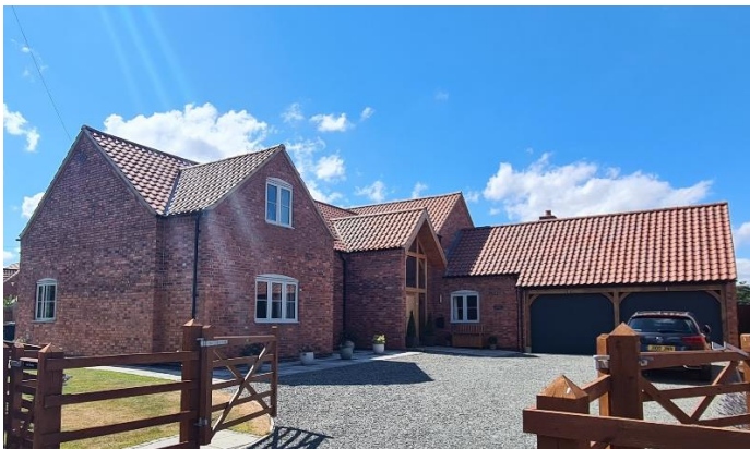
Figure 25 - Swift House, Main Street
