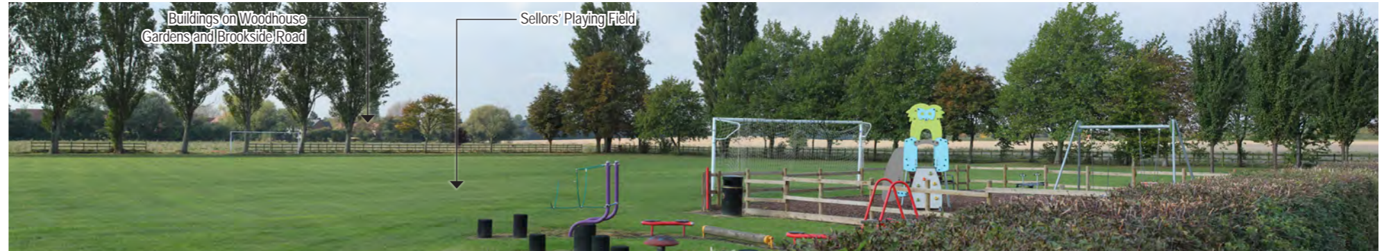
Site Photograph B - This view looks north-west into the site, again from Wilford Road, but a little further south than Photograph A. Sellers Playing Field accounts for the majority of the view, with its boundary lined by an avenue of trees. In the left hand side of the view can be glimpsed buildings on Woodhouse Gardens and Brookside Road.
