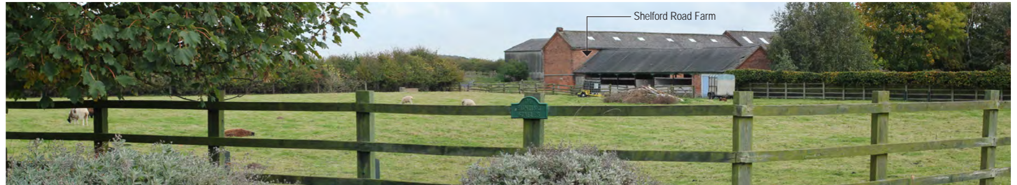
Site Photograph B - This view looks east into the site, again from Shelford Road. Shelford Road Farm features prominently within this view; the brick farm buildings are excluded from the site, but the grey agricultural building beyond falls within the site boundary. The pastoral usage of the site is again apparent from this angle.
