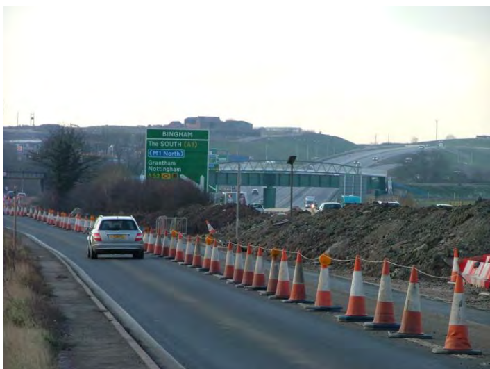
Figure 2.15 Photos of A46. (Old road and new in the back ground)
