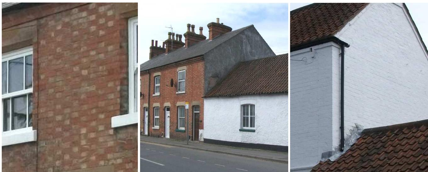
Above (from left to right): different colour shades give Flemish bond brickwork a chequered appearance; a rendered and whitewashed wall stands alongside orange brickwork with ashlar details; white painted brickwork.
