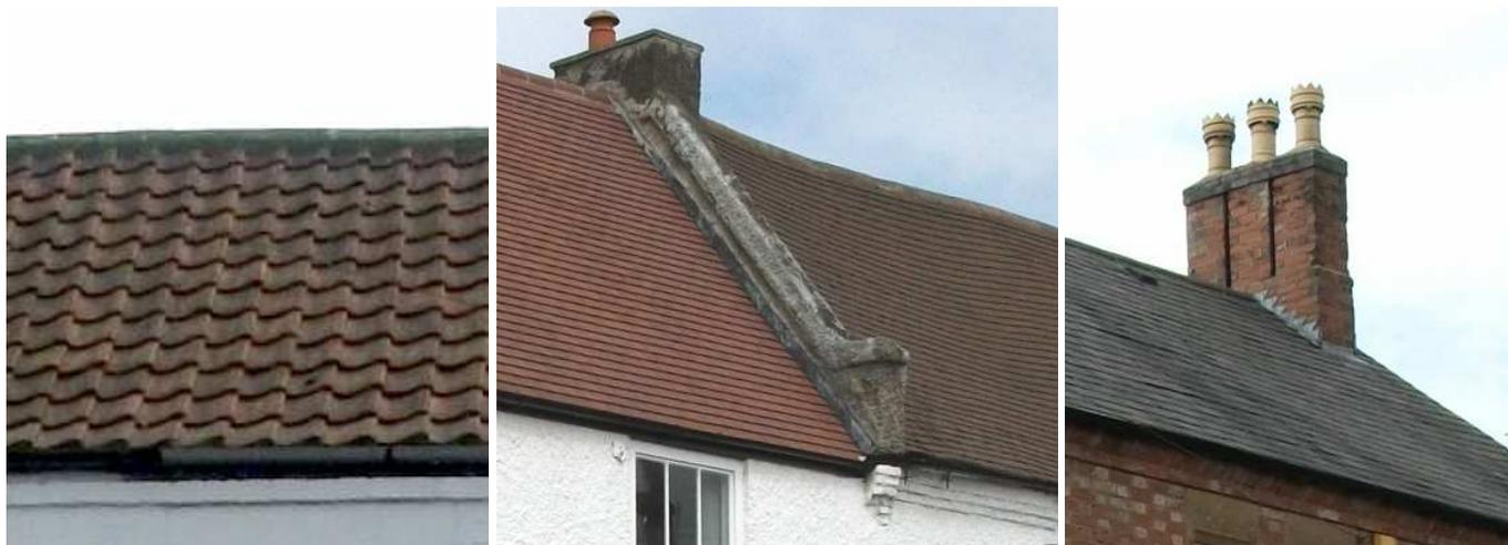
Above (from left to right): Clay pantiles; clay plain tiles and parapet gable; slate roof, brick chimney stack and nineteenth century chimney pots.
