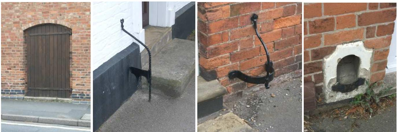
Above (from left to right): timber plank stable door with iron hinges and arched brick lintel; a pair of iron bootscrapers with delicate barley twist arms attached to walls with square headed nails; bootscraper incorporated within a shaped stone surround.
