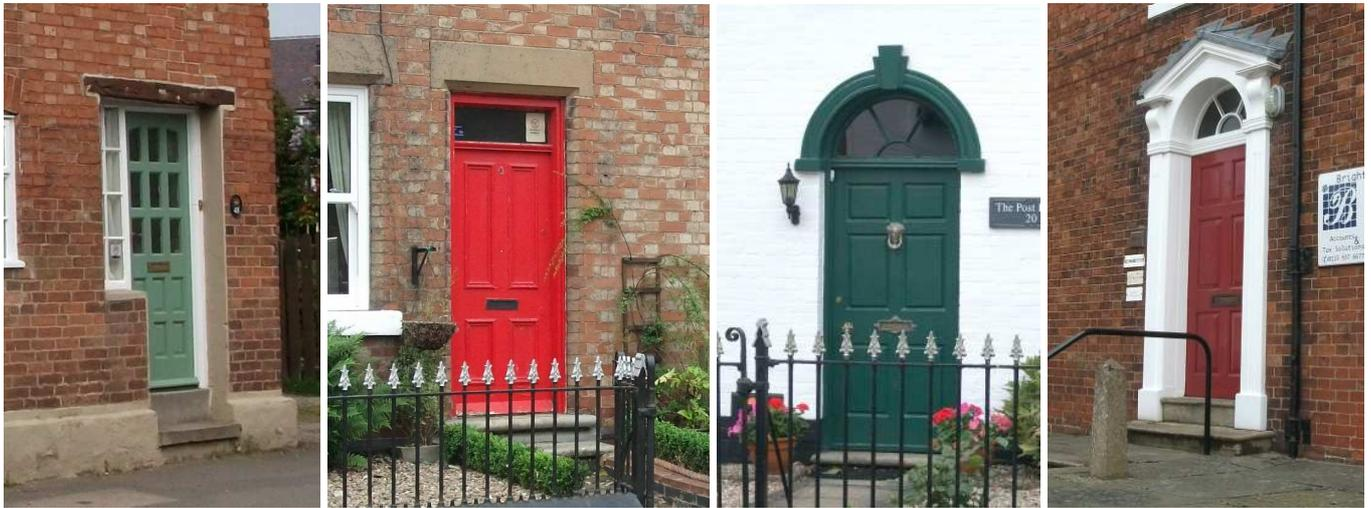
Above (from left to right): timber part glazed door with side window and timber lintel; four panelled door with rectangular overlight and ashlar lintel; six panelled door with fanlight; six panelled door with neo-classical doorcase and fanlight.
