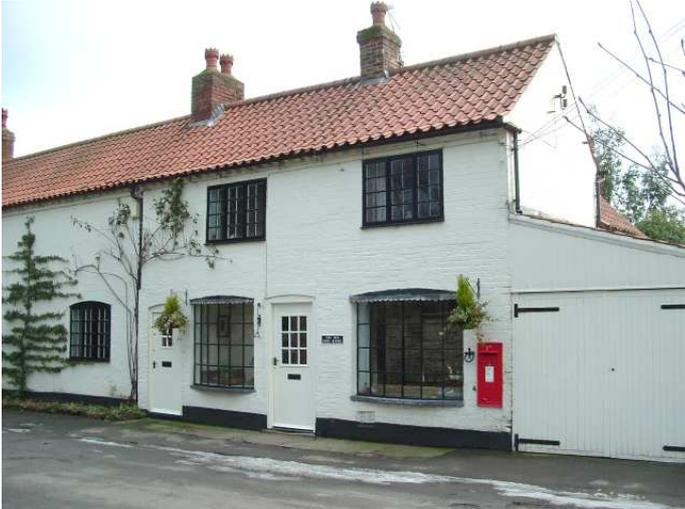
The Old Post Office: bow fronted shop windows on ground floor, part glazed timber door with arched brick lintel, iron letterbox and handle, pantiled roof and white painted brick walls
