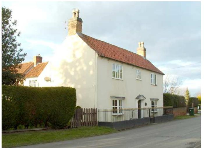
Ivy House Farm: rendered walls, side hung timber casement windows, pediment hood over doorway, pantiled roof and gable chimney stacks.
