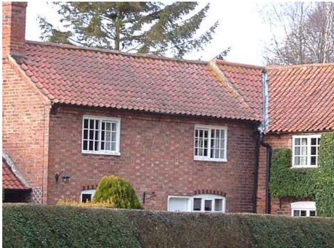
Bumblebee Hall: timber Yorkshire sliding sash windows, Flemish bond patterned brickwork, pantiled roof and decorative arched brick lintels to ground floor window openings.
