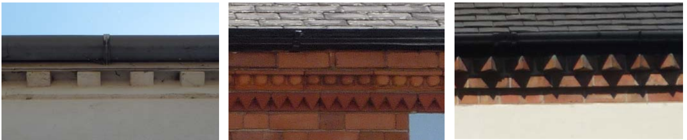
Above: Variations of eaves detailing found within the Conservation Area.
