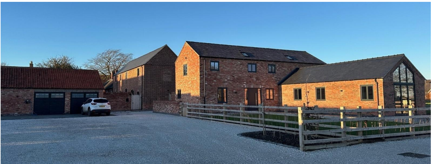
Figure 8 - The mixed conversion and new build scheme at Storeys Yard represents a successful recent development which has restored traditional buildings to use and retained the character of the site
