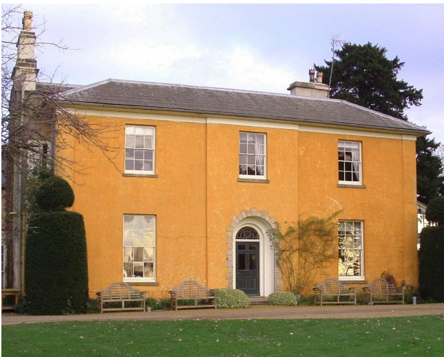
Slate roof, ochre coloured render, symmetrically arranged Georgian sash windows with slim glazing bars and ashlar detailing around the doorway. (Langar Hall).
