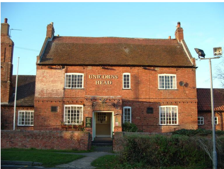
Clay plain tile roof, with parapet gables. Brickwork string course and brick porch. Timber Yorkshire sliding sash windows with segmental headers and arched brick lintels (The Unicorn's Head).
