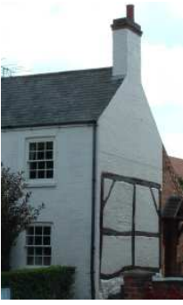
Timber frame revealed on this whitewashed house fronting Main Street.
