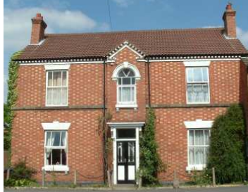
Victorian houses with vertically sliding sash windows, classical style window and door surrounds (above right), dentilated eaves, slate roof (right) and pantile roof (left).
