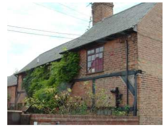
Mid C17 Grade II Listed timber framed cottages with red brick nogging and modern alterations and extensions. Pantile roof (left) and slate roof (right).
