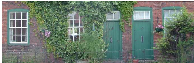
Late C18 glazing bar sash windows and plank doors with glazing bar overlights (Grade II Listed, No.10 Main Street).
