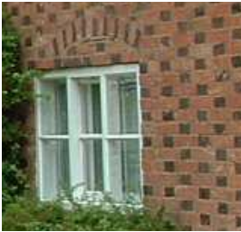
Yorkshire horizontally sliding sash and blue brick chequering.
