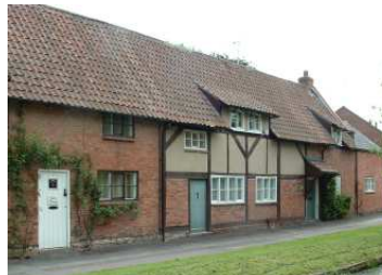
Mid C17 Grade II Listed timber framed cottages with red brick nogging and modern alterations and extensions. Pantile roof (left) and slate roof (right).
