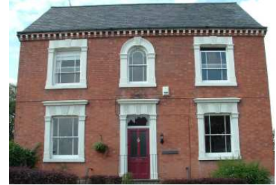
Victorian houses with vertically sliding sash windows, classical style window and door surrounds (above right), dentilated eaves, slate roof (right) and pantile roof (left).
