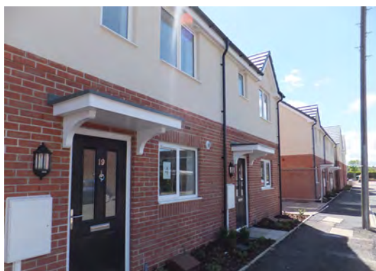
Peatfield Road, Stapleford
