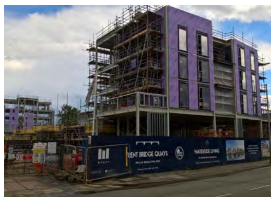
Waterside regeneration, Nottingham
