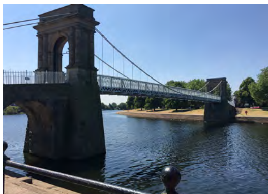
Foot and cycle bridge, River Trent
