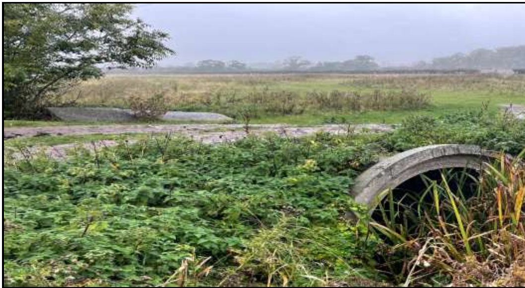
Figure 3.1 – Existing culvert and bridge over Kingston Brook to access Southern Parcel.
