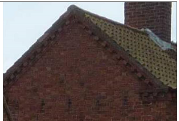
Figure 36 - brick dentil detailing on a farmhouse on Main Street
