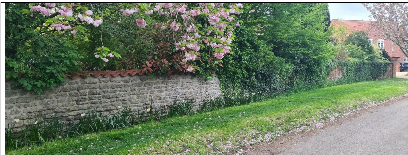
Figure 17 – Stone wall topped with clay pantiles
