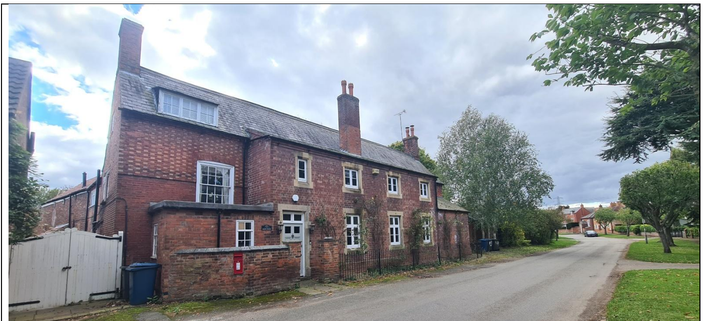
Figure 28 – Beech House with its ashlar heads and cills around the windows and steep roof pitch required for the original thatch.
