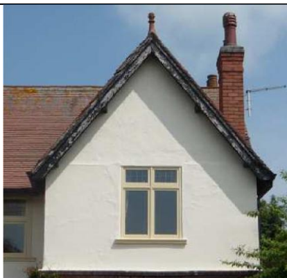
Figure 34 - casement window and finial on the gable end of a house on Main Street
