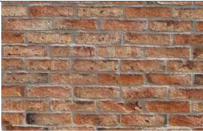
Figure 29 - Stretcher bond brickwork
