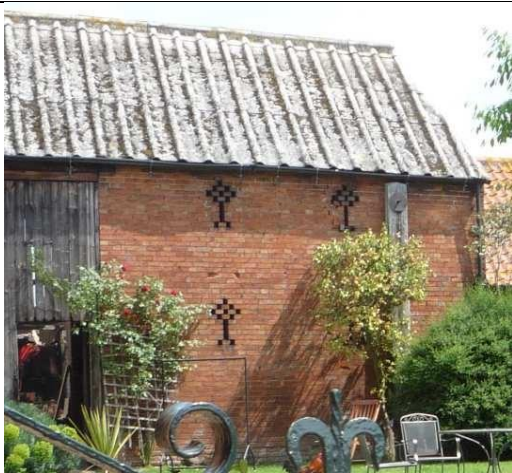
Figure 31 - missing brick patterns in a traditional agricultural building on main Street
