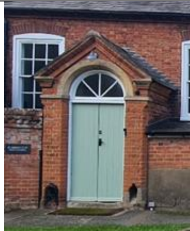
Figure 32 - neo-classical style porch, overlight and vertically sliding sash window on the Wesleyan Chapel on Main Street
