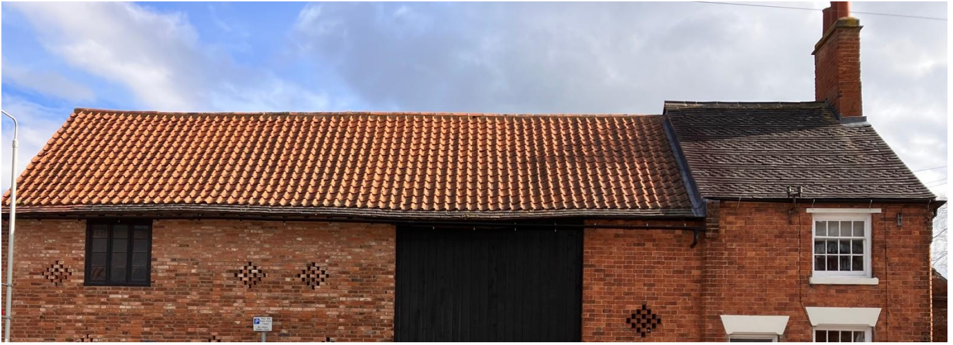
Figure 47 - Clay pantiles and mathematical tiles – Main Street
