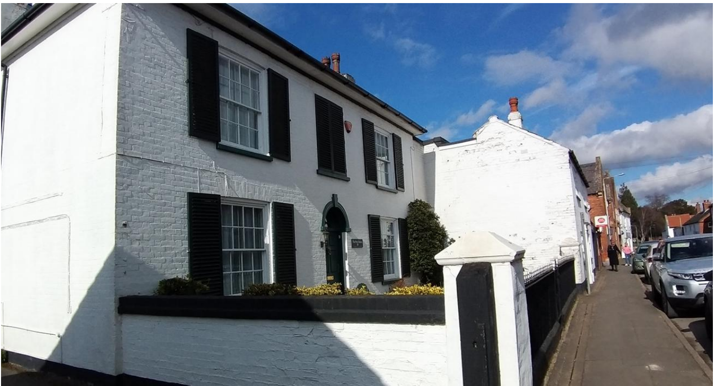
Figure 48 - 16 panes with gauged brick headers
