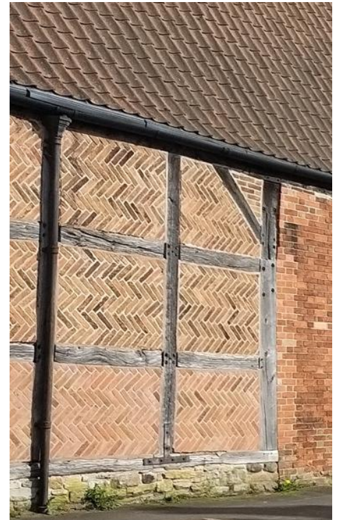
Figure 43 - 18 th century Herringbone brick infill panels on George Martyns Barn, Main Street
