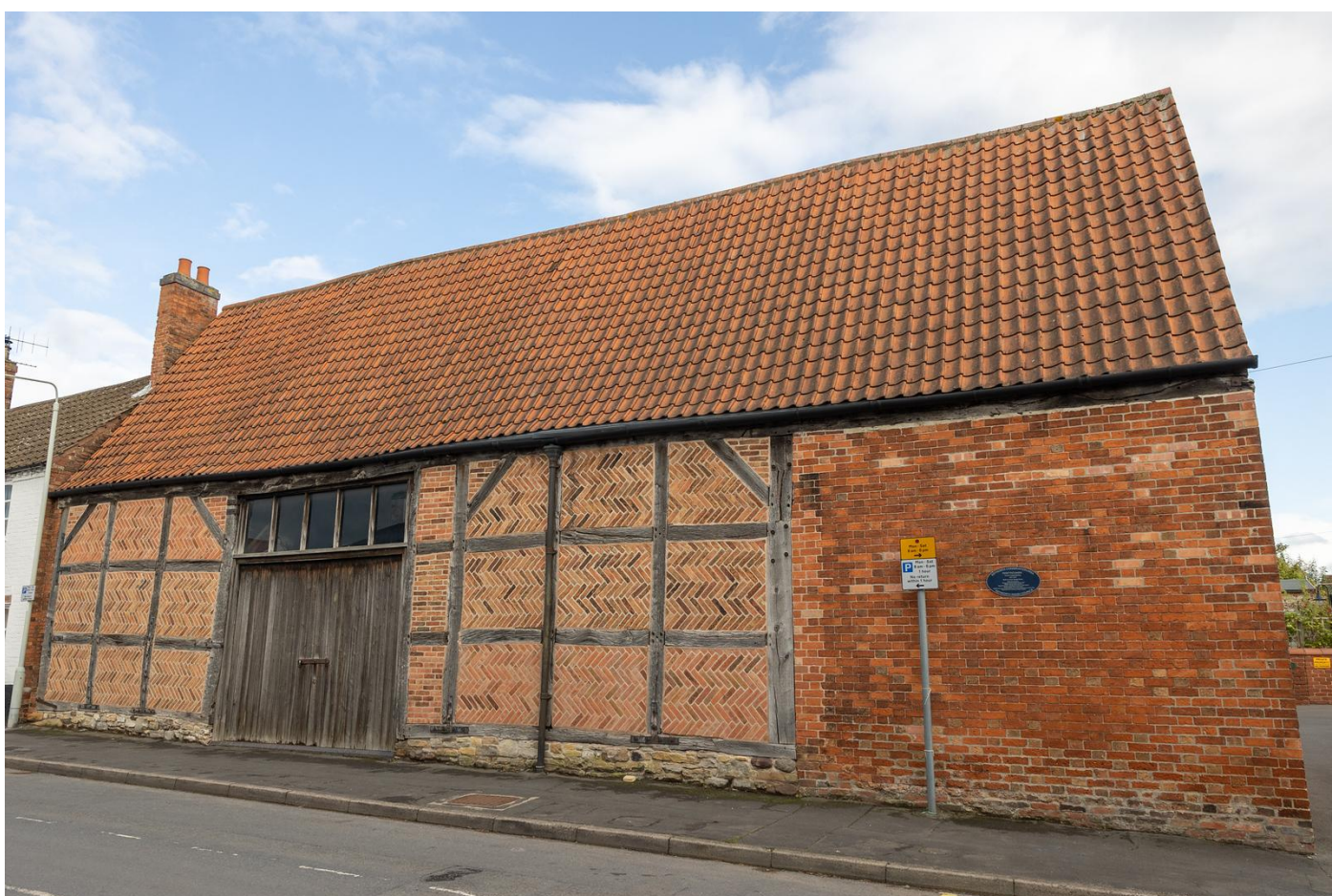
Figure 25 - George Martyn's Barn, Main Street (c1651) (named after farmer George Martyn of Bunny), a 17 th Century timber framed barn with 18 th century herringbone brick infill panels. The frame is built on a Blue Lias rubble plinth and the steep pitch of the pantile roof indicates that it was once thatched.
