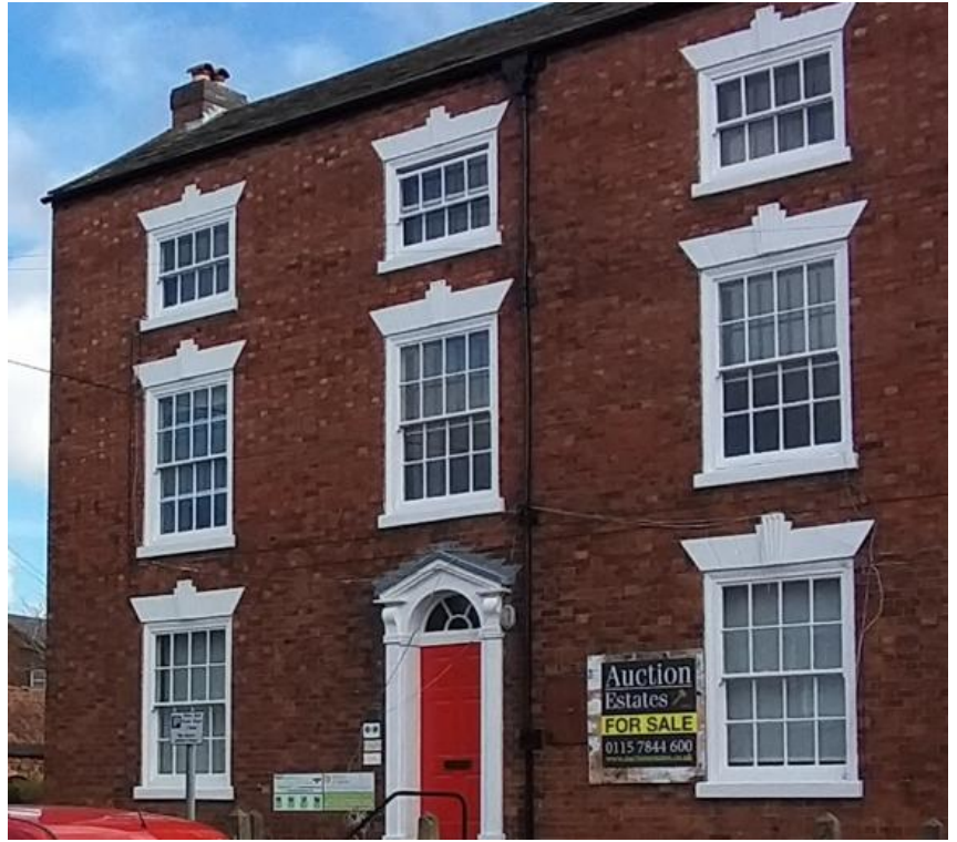
Figure 50 - Hierarchy of panes with wedge lintels and key blocks.
