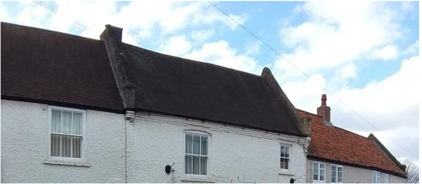
Figure 45 - Plain tiles with parapet gables – possibly indicating former thatch.
