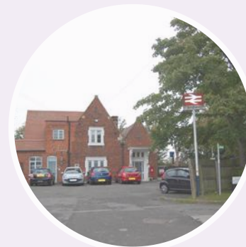
STATION BUILDING: ATTRACTIVE / USED BY OFFICES / LITTLE PARKING AND NO ATTENDANTS
