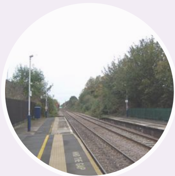
RAILWAY PLATFORMS: UNATTRACTIVE/ POORLY CONNECTED / TOO LOW/ NO TICKET MACHINE
