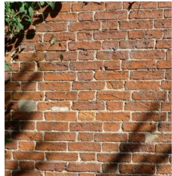
FIGURE 24: EXAMPLE OF TRADITIONAL LIME POINTING
