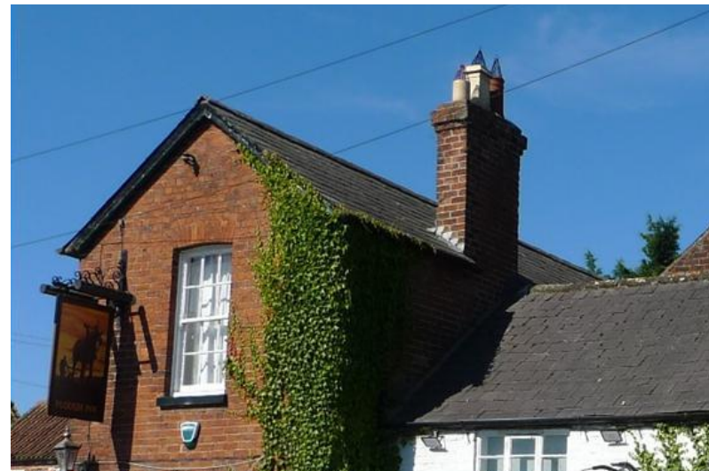
FIGURE 15: EXAMPLE OF A SLATE ROOF ON THE PLOUGH INN
