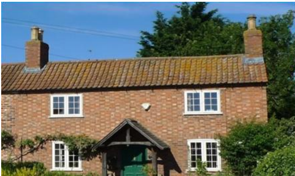
FIGURE 16: EXAMPLE OF A PANTILE ROOF
