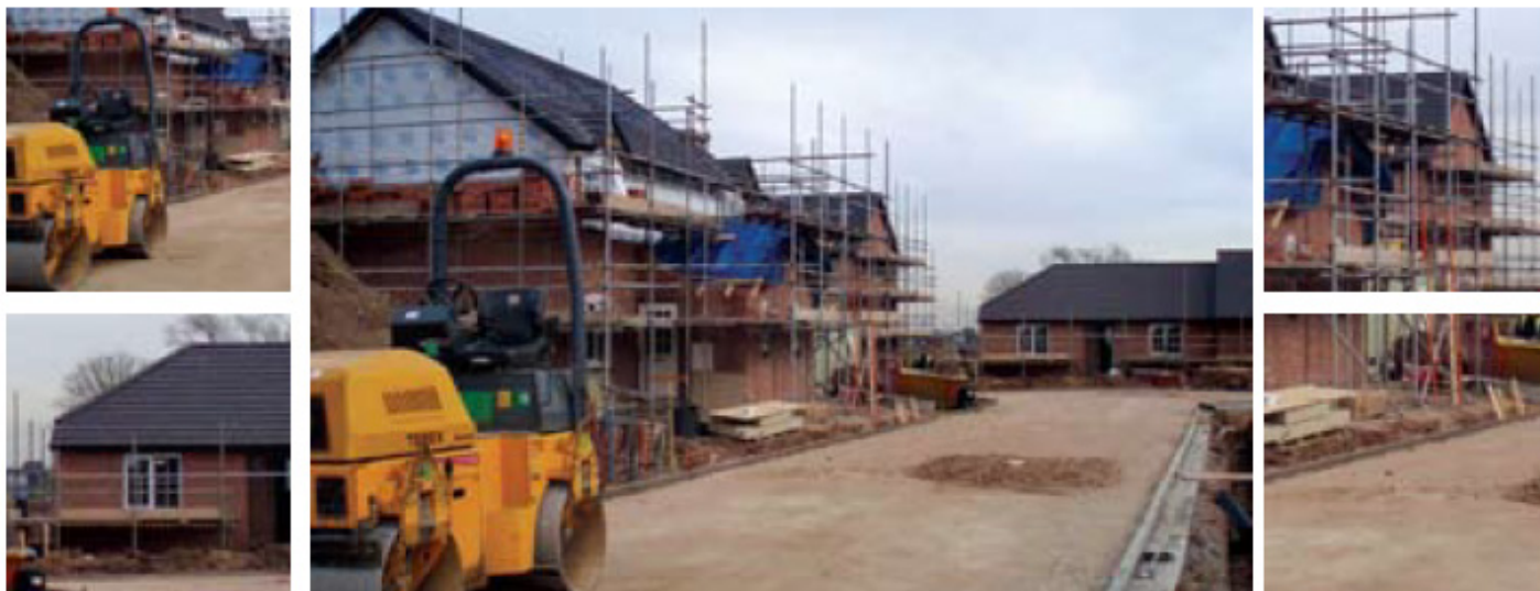
Affordable housing under construction in East Bridgford
