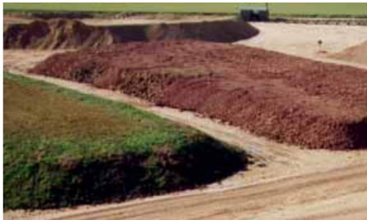
Clearly defined stockpiling of different soil materials
