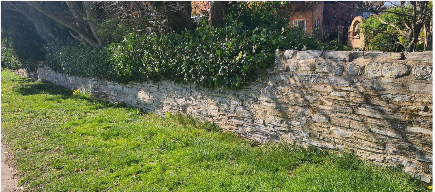
Figure 13 – Lias Stone Wall along Sutton Lane
