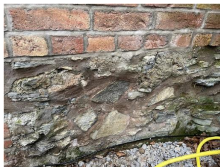
Figure 26 - C19 Brick on older stone foundations
