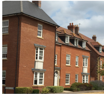
Prominent corner building with windows on both front and side elevations.
