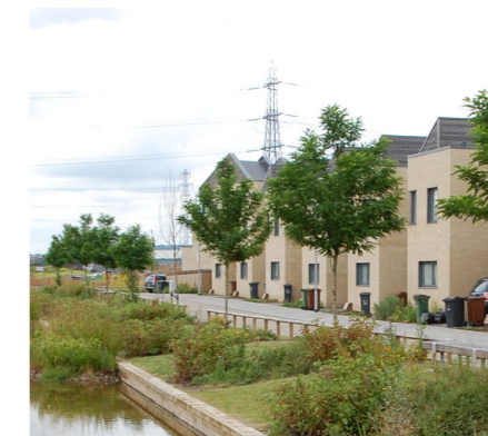
Consistent street scene with 2 storey dwellings overlooking water feature.
