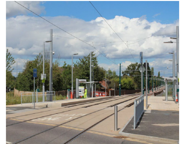
Nottingham Express Transit (NET) Ruddington Lane stop within 10 minutes cycling distance of the site
