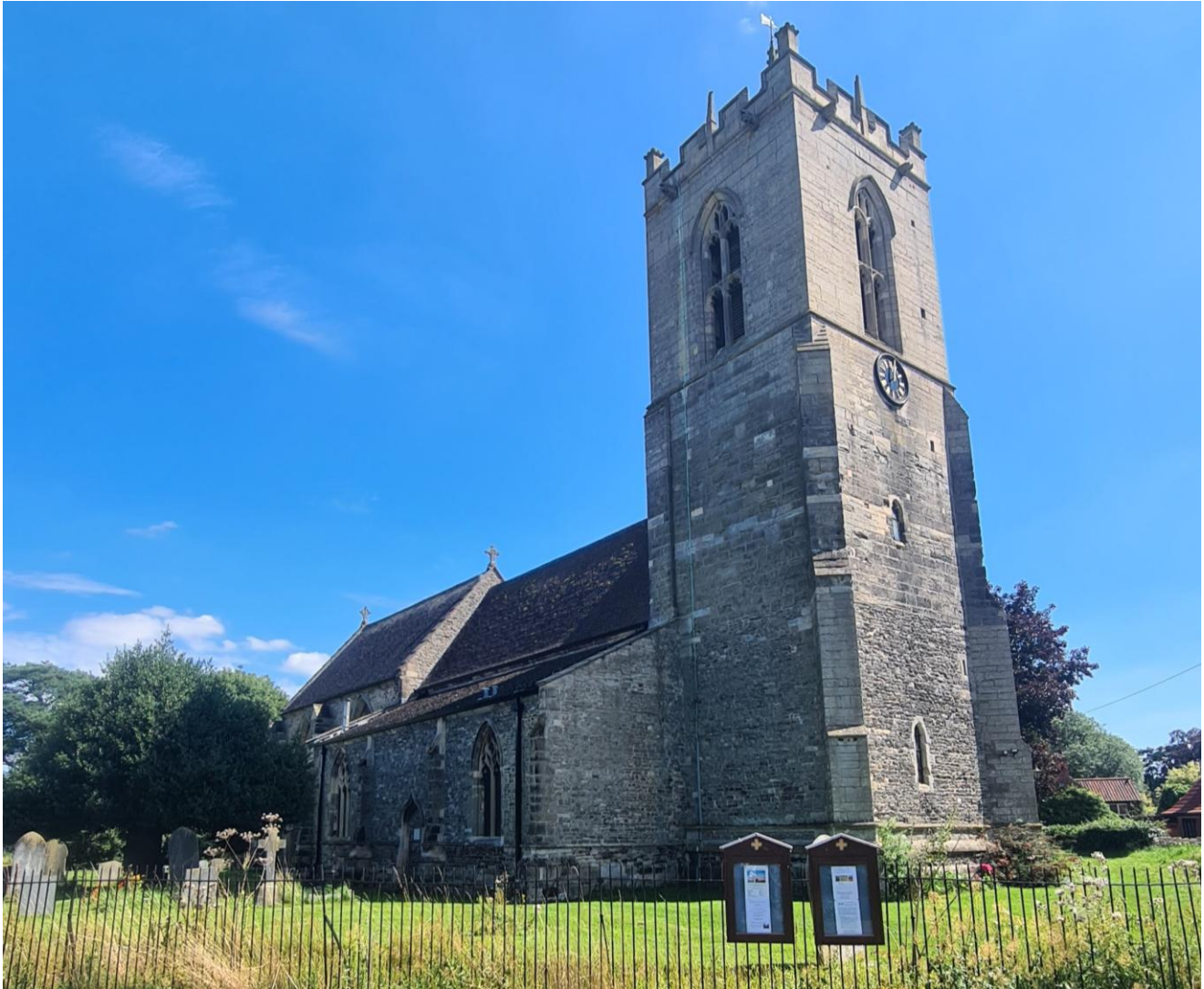
Figure 25 – St Mary's Church – Screveton Road
