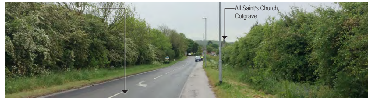
Site Photograph B - This view looks southerly along Main Road and demonstrates both the separation of the site from the main settlement edge, as well as the overall character. In the background of the view can be seen the spire of All Saint's Church, which sits in the north of Colgrave itself.
