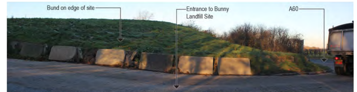
Site Photograph C - This view looks directly into the site, from the entrance to Bunny Landfill Site - just off the A60. The bund visible in the foreground is part of the site.
