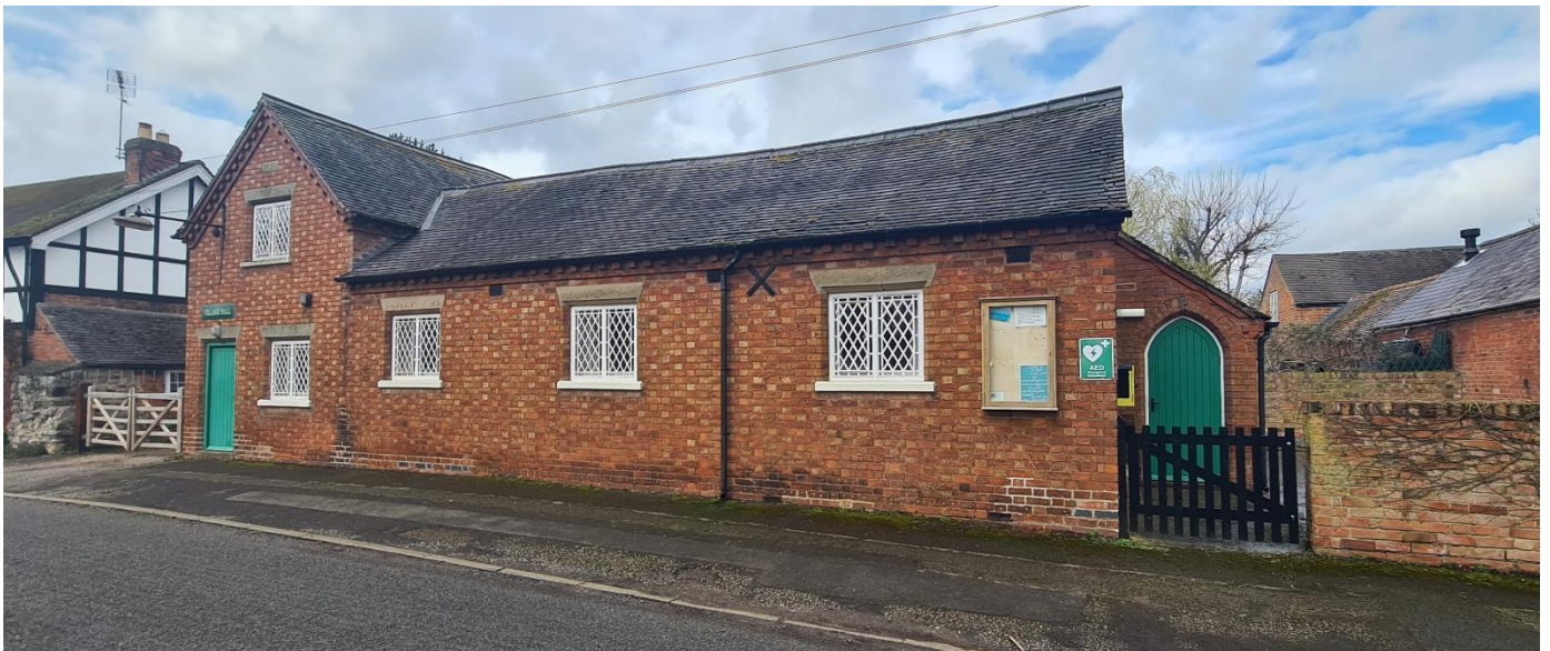
Figure 15 – Village Hall (built 1850)
