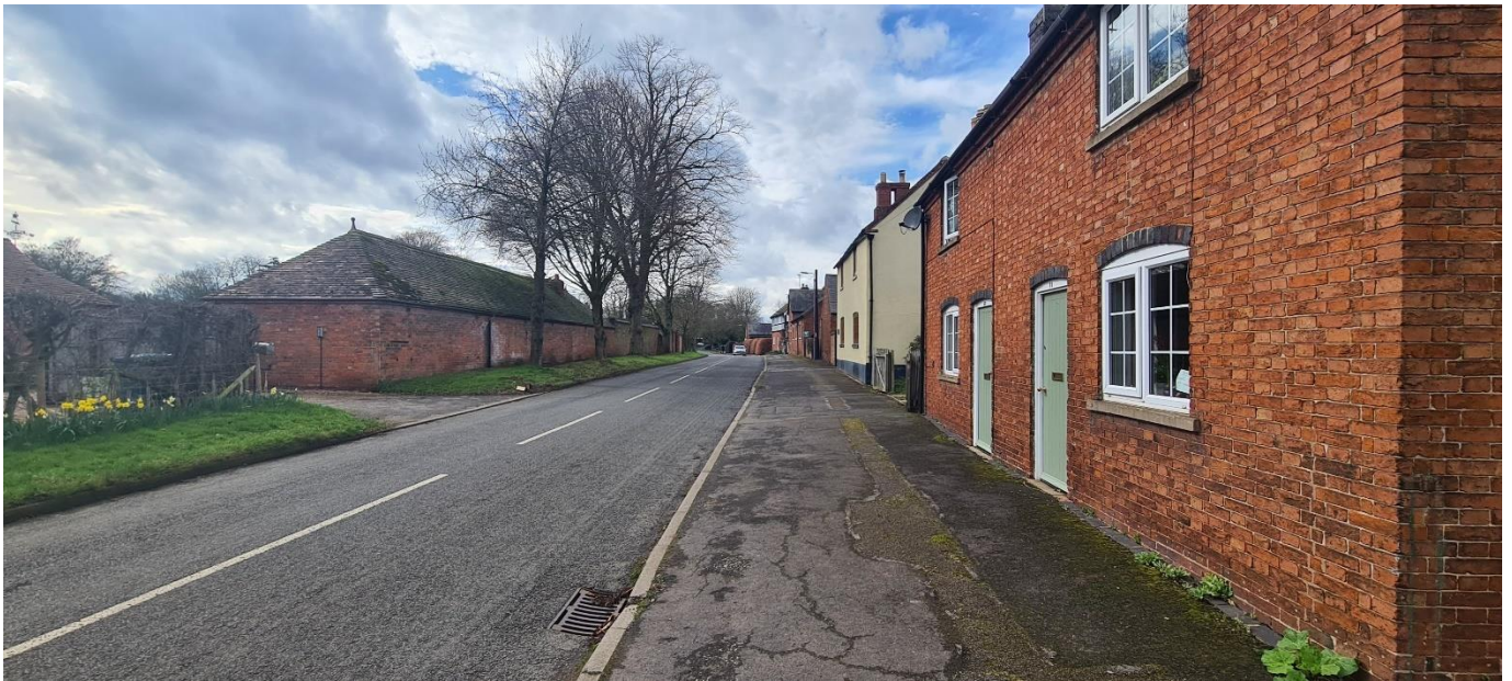
Figure 11 View along Main Street from the West looking towards the East
