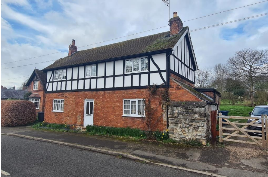
Figure 13 – Former Post Office, which has partial stone foundations was reconstructed with a mock, half-timbered style.
