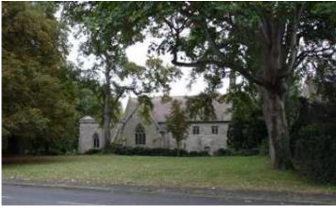
Figure 8 - Open Space in front of St Helena's Church
