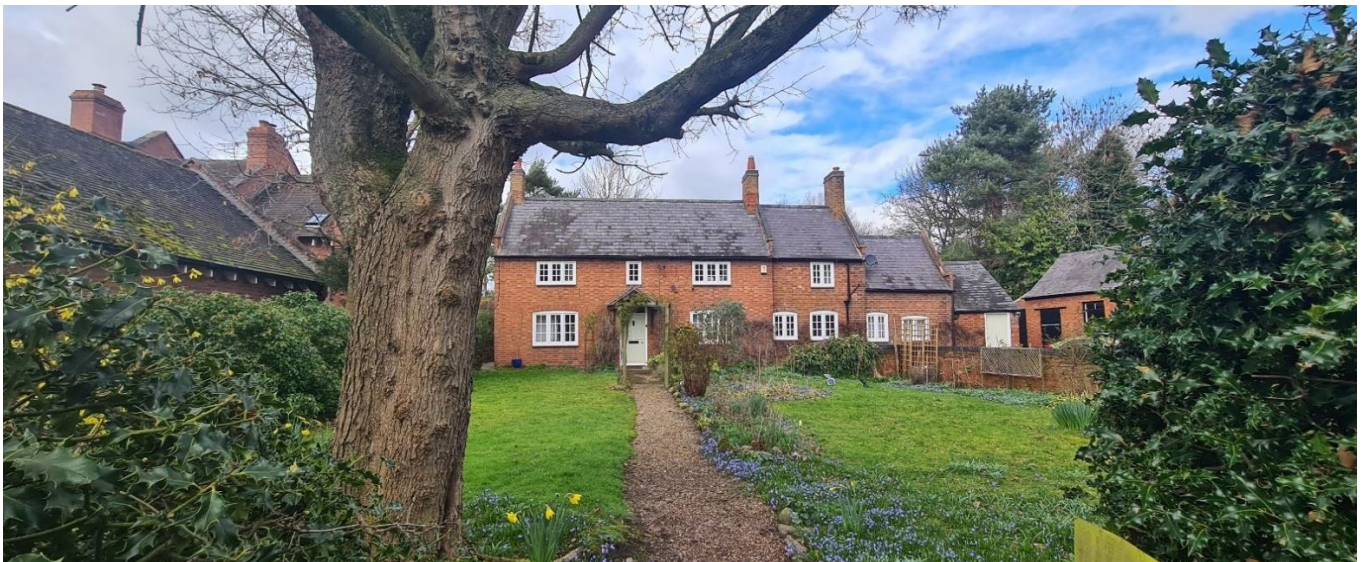
Figure 18 - No. 55 Main Street, West Leake (Grade II Listed)
