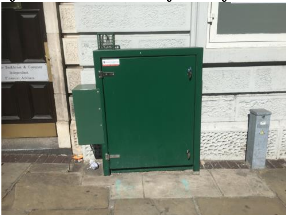
Figure 4 – Photo of AQMA1 Trent Bridge Monitoring Station
