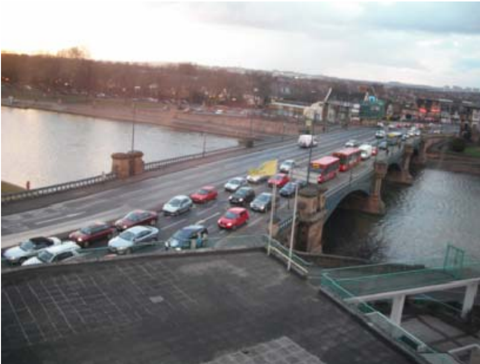
Photo of Trent Bridge showing peak flow out of the city
