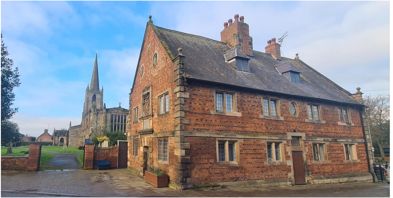
Figure 30 – Former Schoolhouse and St Mary's Church
