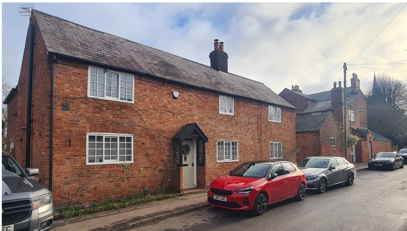
Figure 34 – 10 and 12 Moor Lane
