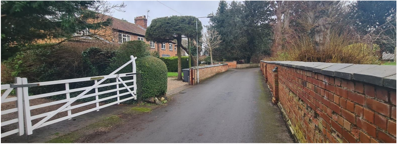
Figure 18 – 5 bar curved heel timber gate (left) and wall
