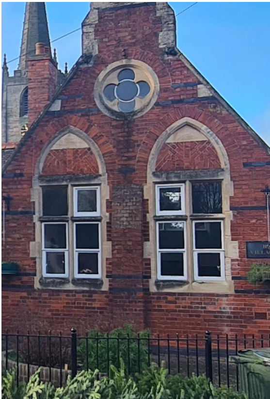
Figure 27 – Brick detailing on the former School
