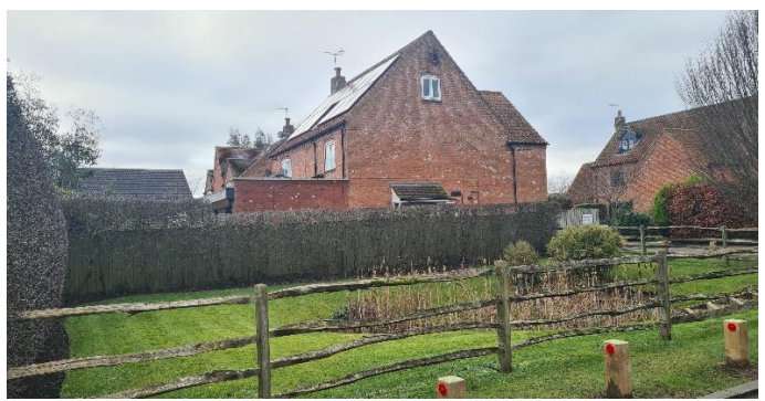
Figure 15 – Wooden fencing surrounding the attenuation pond
