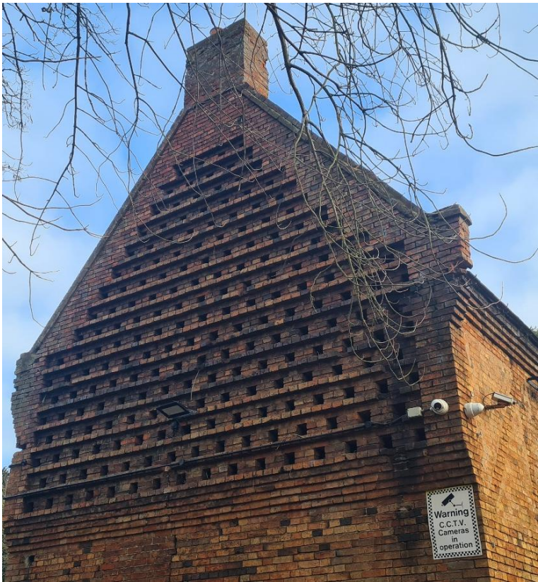
Figure 28 – Brick details on the former pigeoncote
