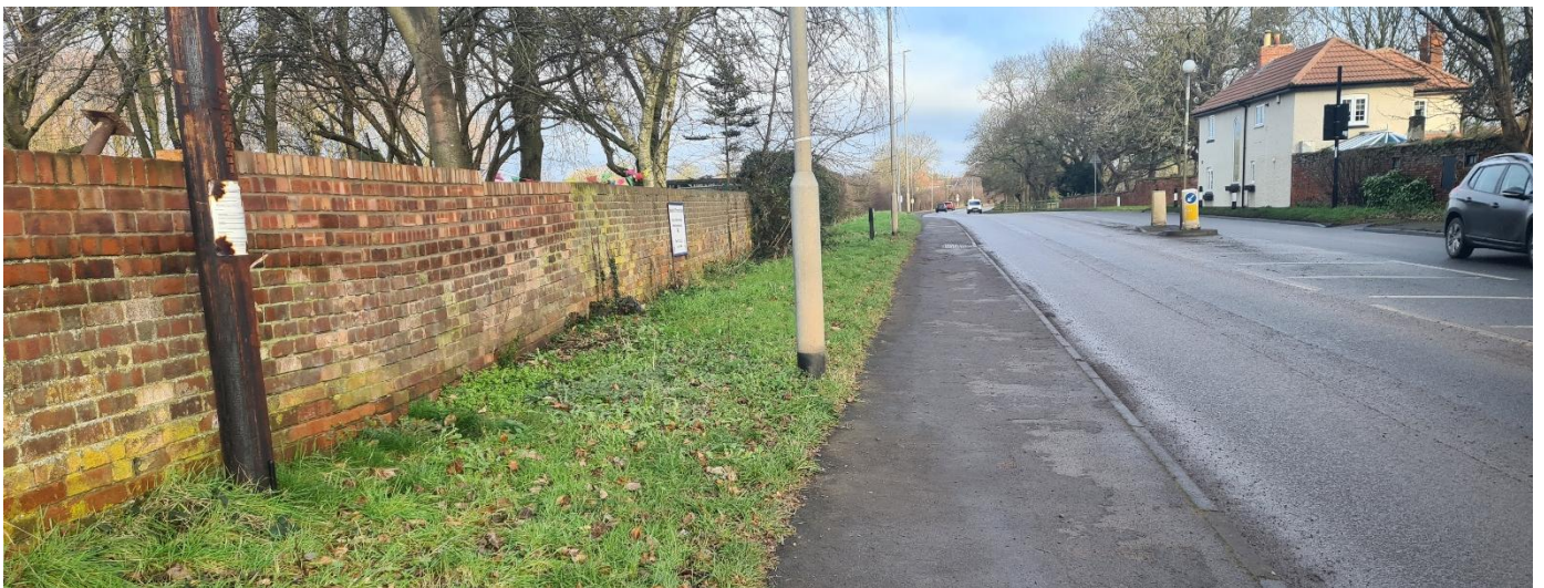
Figure 17 – Wall Along Loughborough Road to the North
