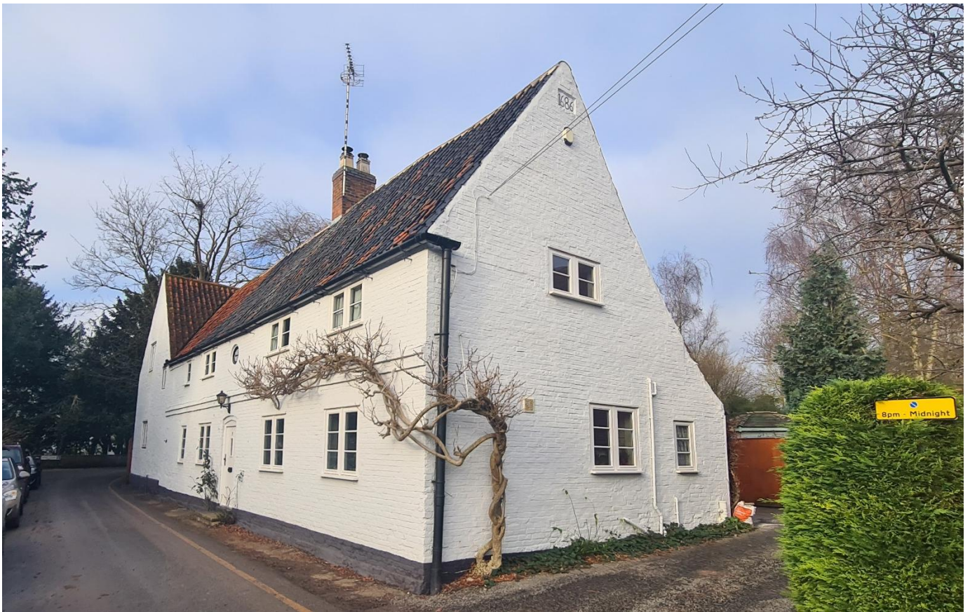
Figure 33 – The White House (Grade II)
