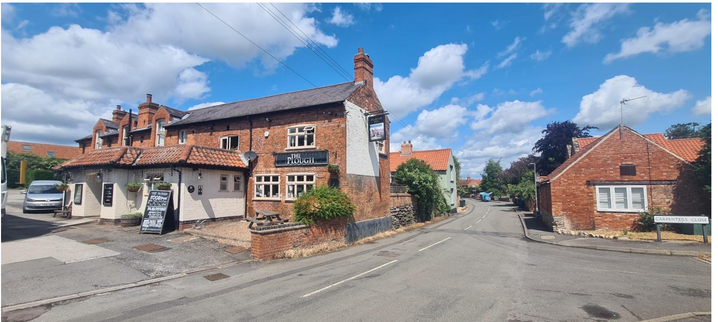
Figure 18 – The Plough Inn Public House
