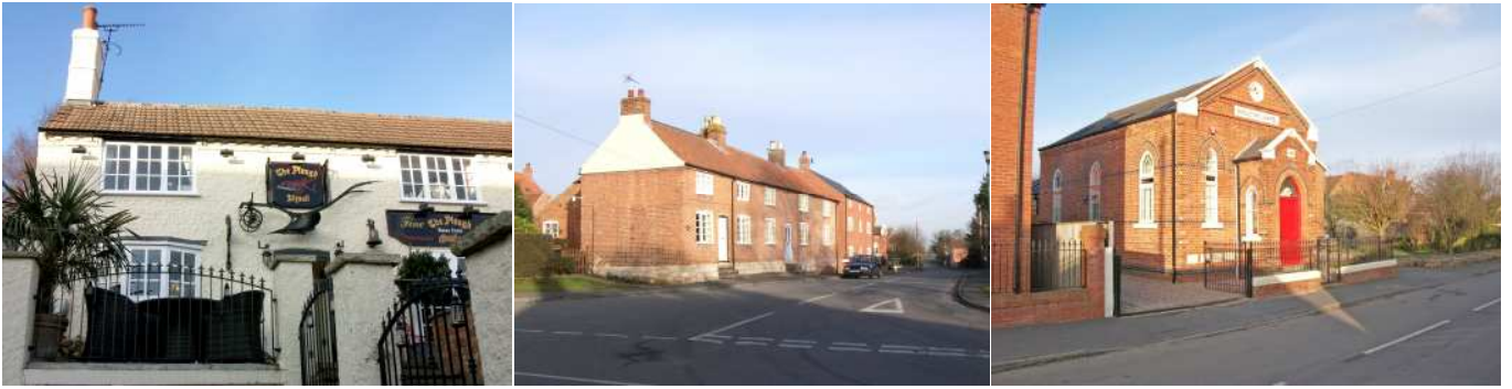
From left to right: The Plough Inn Public House on Keyworth Road is an important community facility; Homestead and Brynstone Cottage in their prominent position at the junction of Main Street and Widmerpool Road; the Wesleyan Chapel of 1881 was built to replace an earlier Victorian structure. It is now a private dwelling.
