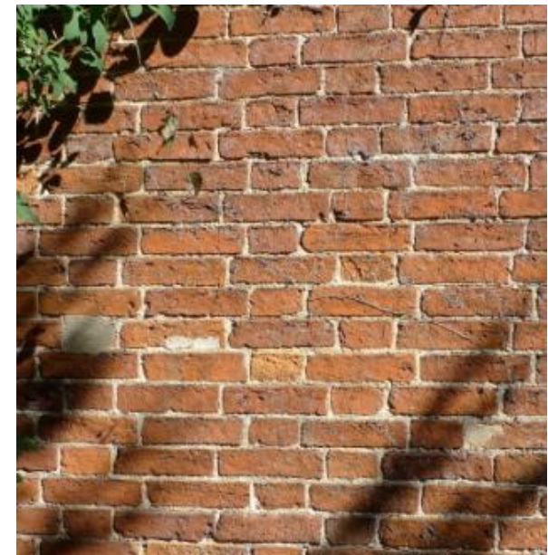
FIGURE 24: EXAMPLE OF TRADITIONAL LIME POINTING
