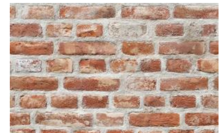
FIGURE 23: EXAMPLE OF POOR POINTING WITH WIDE JOINTS AND MORTAR SMEARED OVER THE FACE OF THE BRICKS
