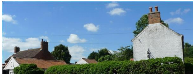
FIGURE 17: EXAMPLE OF A 45 PITCH GABLE
