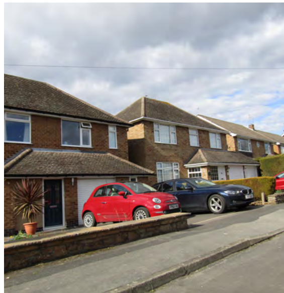
Mix of hipped and front to rear pitched roofs
