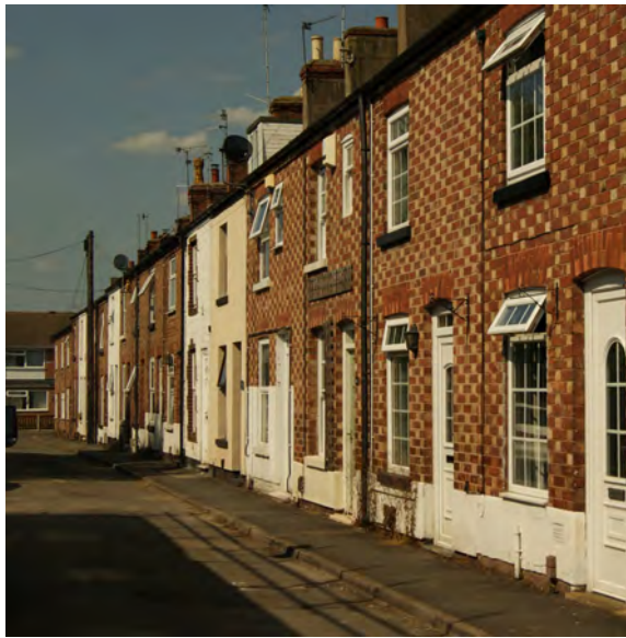
Mid-19th century terraces with a narrow plot width and no front boundary
