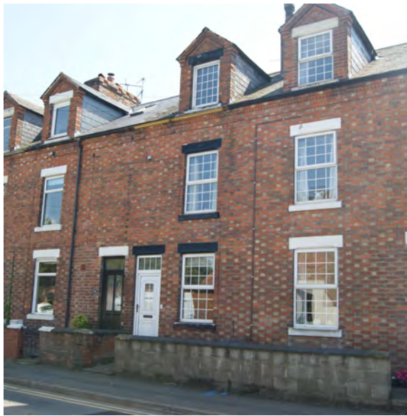
The 2.5 storey dwellings along Kirk Lane use red brick
