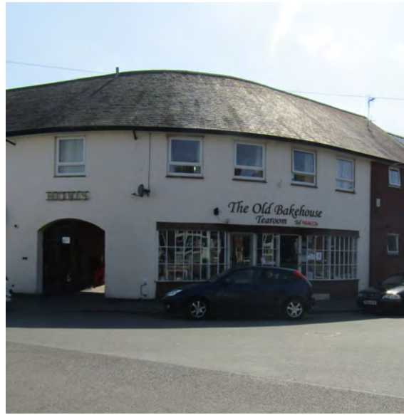
Corner turning terraced properties on Church Street
