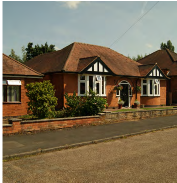
Boundaries are mostly well defined by low brick walls, however some boundaries have been replaced by driveways
