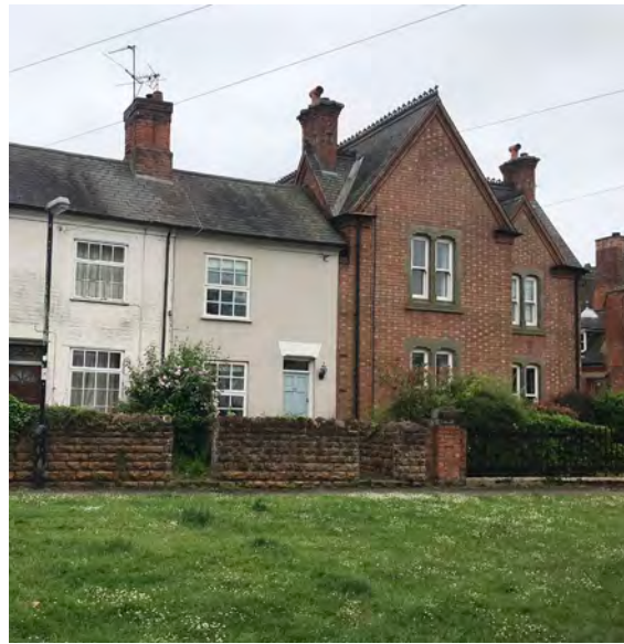
Header building with chequered brickwork in a Flemish bond
