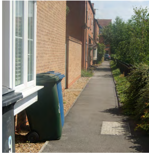
The sustainable urban drainage system is located to the front some semi-detached properties
