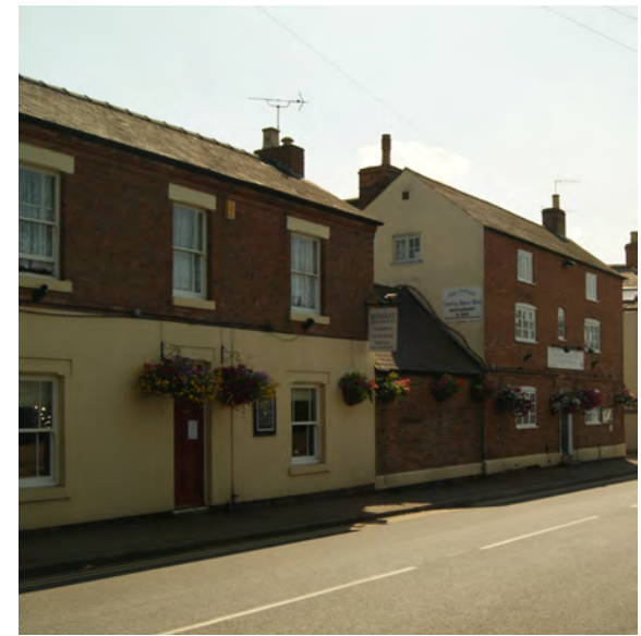
Use of red brick and white render with stone decoration around the windows is common in this area
