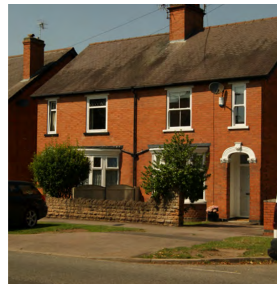
The use of red brick is consistent in this area with decorative door arches, boundaries are defined with a low wall
