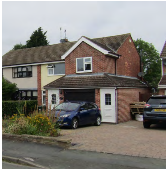
Extensions and alterations forward of the building line contribute towards the character of the area
