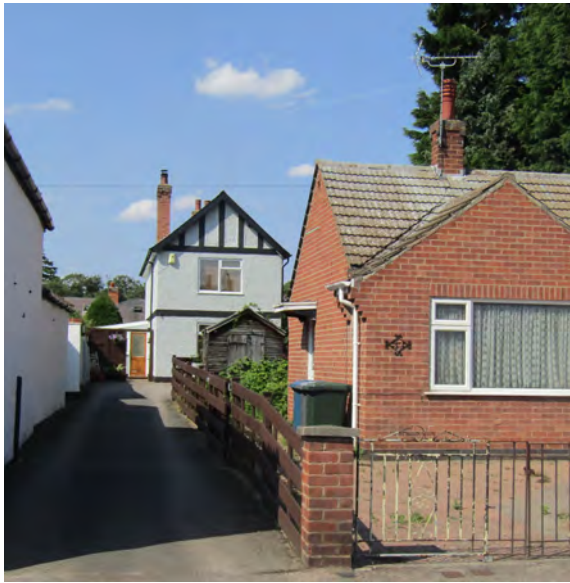
Typical example of backland development along Distillery Street
