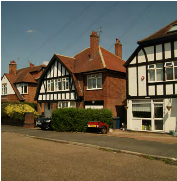
Common materials used are red brick, white render and black and white half-timber
