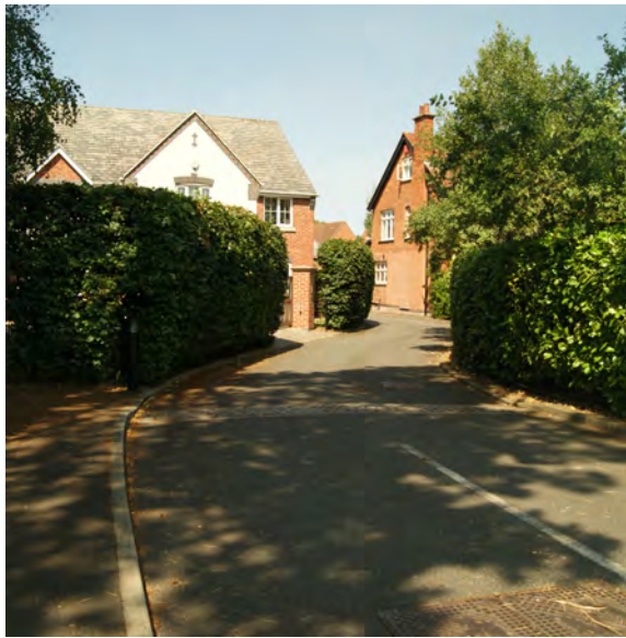
The contemporary backland development off Kirk Lane is accessed through a narrow road that has no pavement
