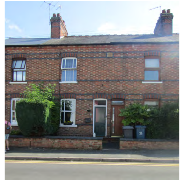
Flemish bond, red and brown brick detailing
