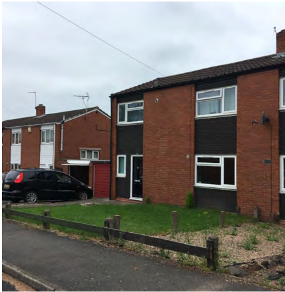
Red brick terraced dwelling with timber cladding
