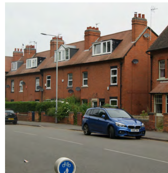
Victorian 2.5 to 3 storey terraced housing to the east of the character area
