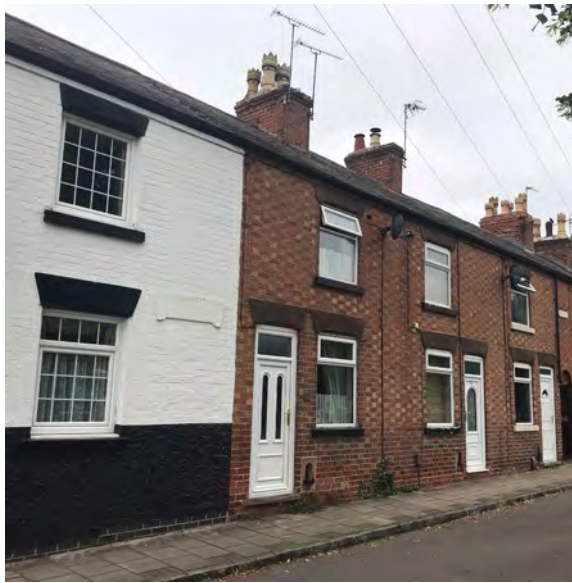
Terraces without front boundaries, providing an example of white painted brick
