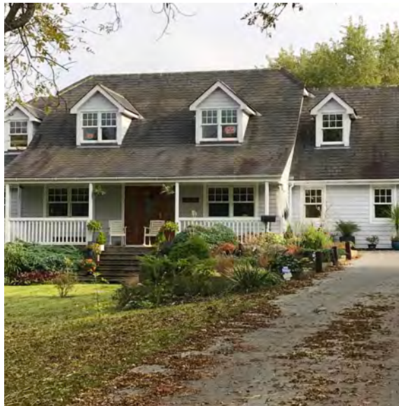
Gabled dormers and timber weather boarding
