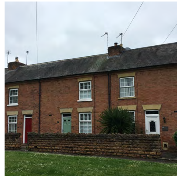
Terraces fronting The Green, set back behind Bulwell stone walled boundaries, with stone lintels and sills
