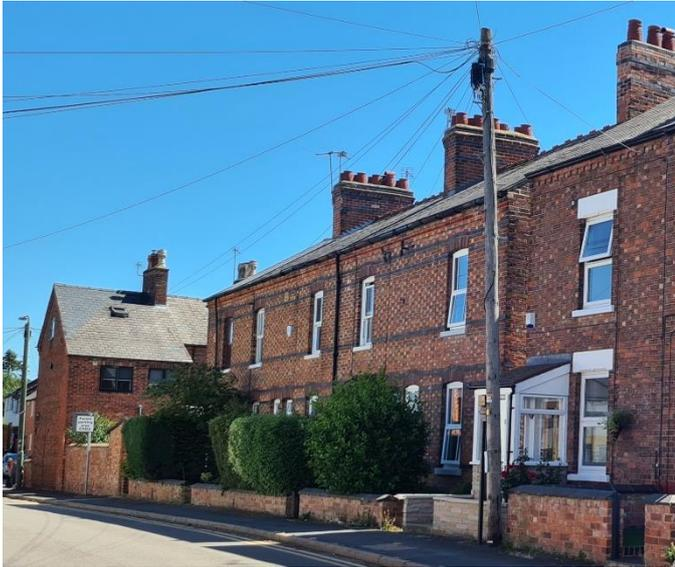
Figure 9 – Low to medium height walls with triangular coping
