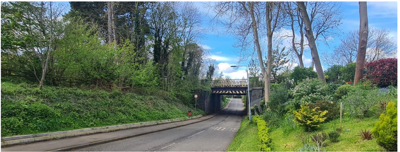
Figure 19 – East Leake bridge and former platform station (zone 2)
