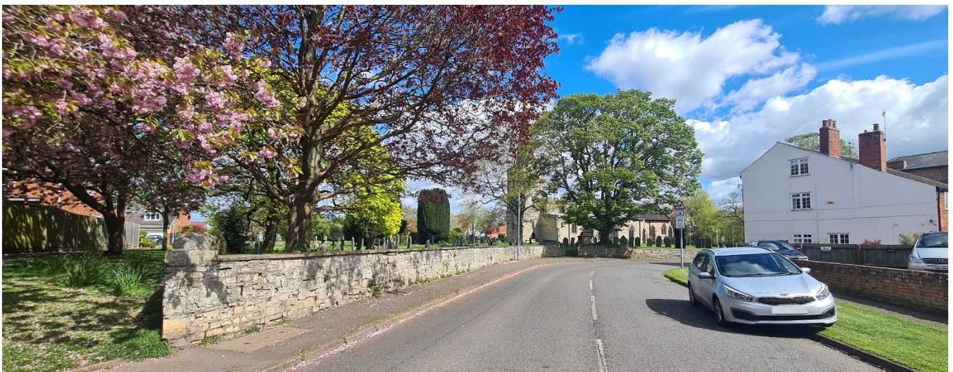
Figure 18 - Stone Wall at the Church and Brick Wall Opposite (Zone 1)
