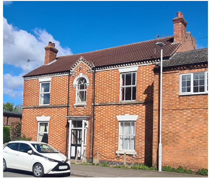
Figure 26 - Victorian house with vertically sliding sash windows, dentilated eaves, pantile roof and Flemish bond brickwork (Zone 3)
