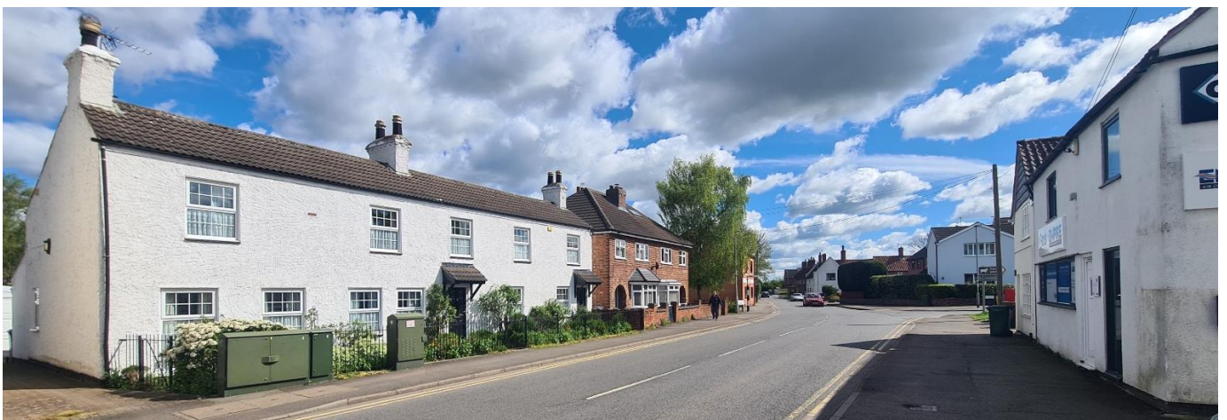
Figure 27 – Rendered and painted properties along main street (Zone 3).
