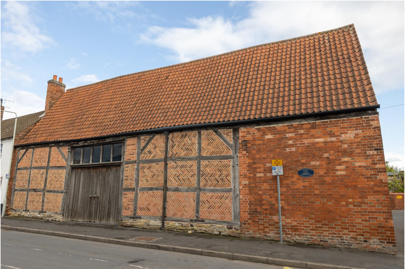
George Martyns Barn, Main Street (c1651) (named after farmer George Martyn of Bunny), a 17 th Century timber framed barn with 18 th century herringbone brick infill panels. The frame is built on a Blue Lias rubble plinth and the steep pitch of the pantile roof indicates that it was once thatched.
