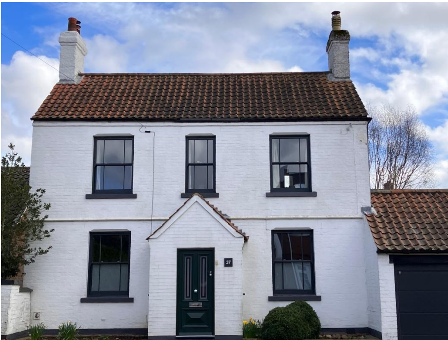
Symmetrical light timber sash windows in painted brick with pantile roof – 37 Main Street
