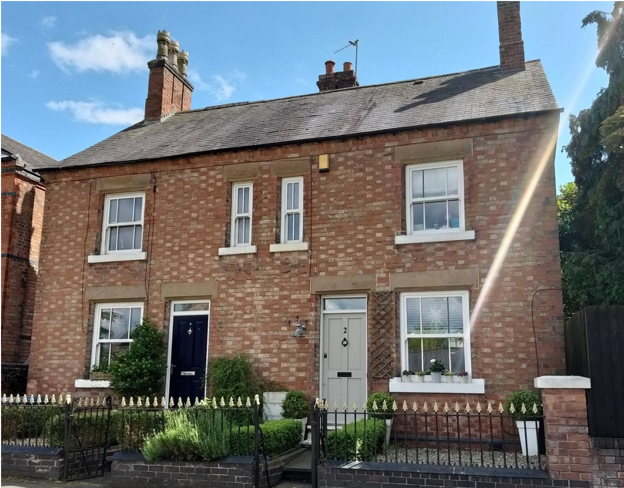
2 and 4 Selby Lane- Flemish Bond brickwork is common in the centre of the village. The use of light headers gives a pleasant chequered appearance here.
