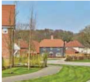
High quality surface materials and tree planting to be a dominant feature.
