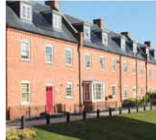
Formal street scene with consistent dormer windows and chimneys.
