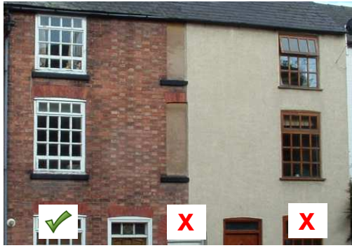
The dramatic effects that inappropriate alterations can have (windows filled-in, brickwork covered with render, brown glazing bars instead of white).
