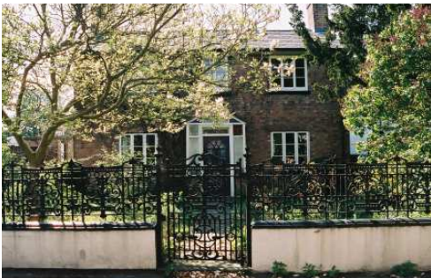
Original boundary wall and railings are of equal importance to the historic building behind.
