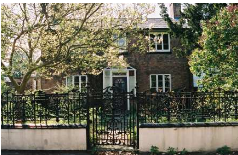
Original boundary wall and railings are of equal importance to the historic building behind. (example taken from East Bridgford).
