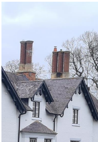
Figure 29 – Barge Boards and Chimney Stacks at The Gables, Church Street, (Zone 1)
