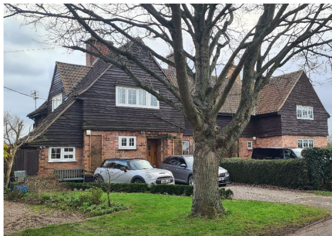
Figure 34 – Timber Cladding at 5 and 7 Conery Lane, (Zone 1)
