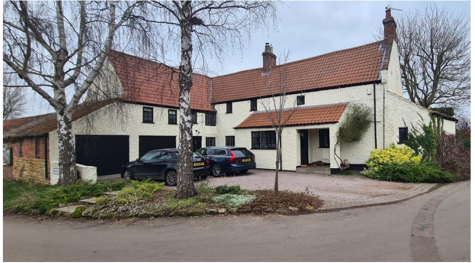
Figure 20 - Tyler's Cottage, Sunbeam Street, (Zone 1)
