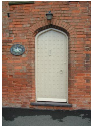
Lead capped coping at No.2 Church Street (left), battened and studded door in the Old Vicarage wall (centre) and timber gate at No.12 Moor Lane (right).
