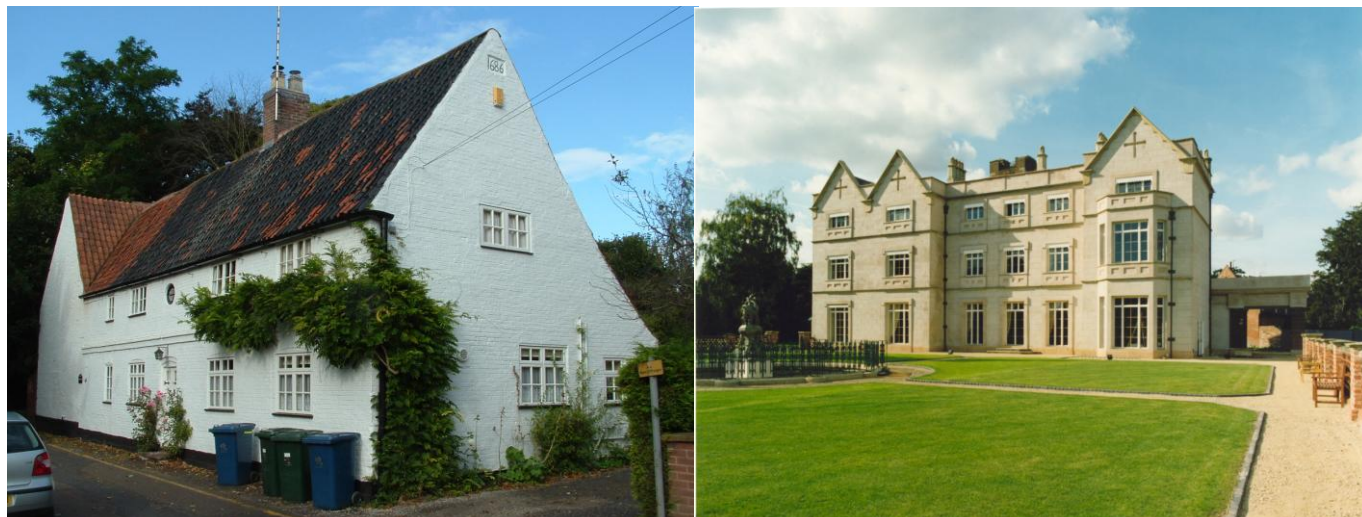
The White House (Grade II) and Bunny Hall (Grade I).
