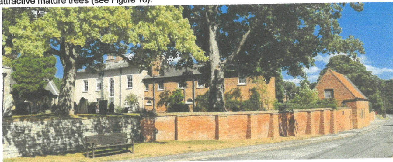
Figure 16 - Mature Trees in Church Yard and Retaining Wall
