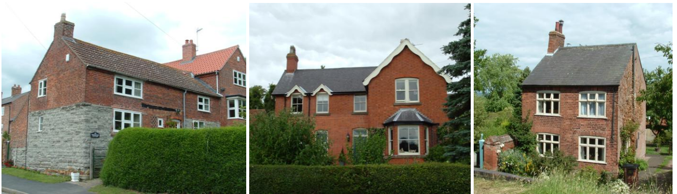
Left: Greystone Cottage, Station Road displays various phases of construction. It has local blue lias stone walls with brickwork in an English garden wall bond above. Centre: Orchard Lea, Station Road, a fine example of a late Victorian villa with four pane timber sash windows, moulded timber barge boards, Flemish bond brickwork and a Welsh slate roof. Right: 19 th century cottage on Rectory Drive with a random brick bond and tripartite timber casement windows under arched brick lintels.
