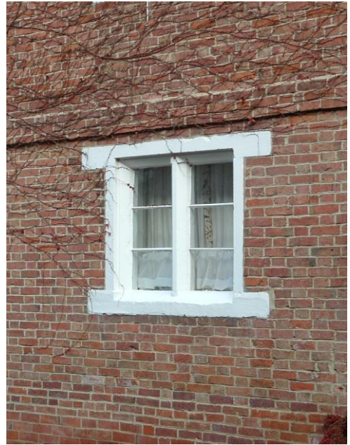
Single mullioned ashlar casement window with puddle wrought iron glazing bars
