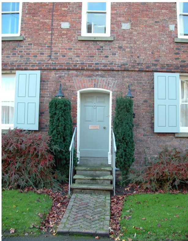
Decorative red and blue brick string course, sliding sash windows and panelled timber door with arched brick lintel.
