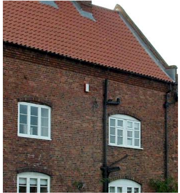
Orange clay pantile roof with parapet gable, decorative brick eaves, arched brick lintels and timber casement windows with segmental headers.
