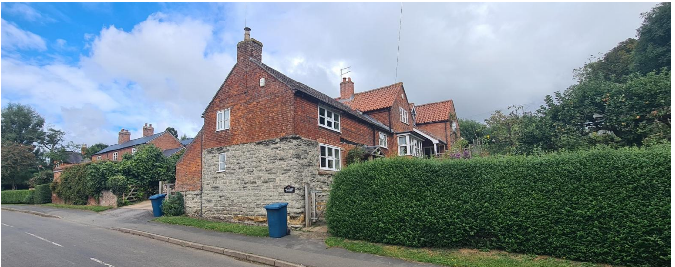
Figure 27 - Greystone Cottage, Station Road. Shows various phases of construction. It has local blue lias stone walls with brickwork in an English garden wall bond above.
